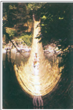
Figure 6.7 : Rope Bridge (Arunachal Pradesh)
