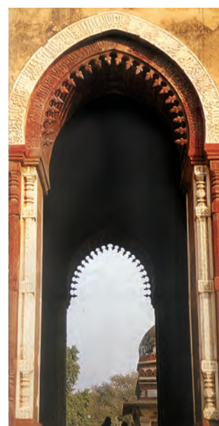
Fig. 5b True arch; detail from the Alai Darwaza (early fourteenth century). Quwwat al-Islam mosque, Delhi.
